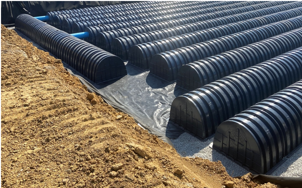
Figure 1: A Main Header Row is shown on geotextile fabric on the top left of the image and is connected to the system by cross-connection pipes.
